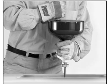
**Tips:** If you cannot get the cable through a trap, unscrew the clean-out plug. Be sure to put a pan under the plug before unscrewing. Insert cable into clean-out opening.
