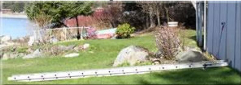
**First** - lay extension ladder flat on its back with feet of the ladder butted up against building's wall and the fly side down.
