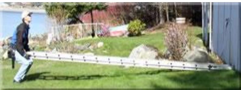
**Second** - lift ladder's top while pushing forward to maintain pressure against building's wall. \*Don't perform ladder work if you are not mentally or physically capable of safely accomplishing the work. \*Lift with your legs, not your back.
